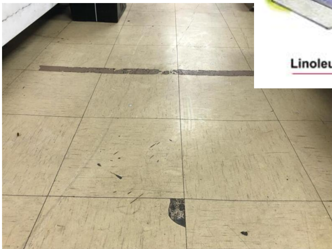
Asbestos Vinyl Floor Tiles Gallery
